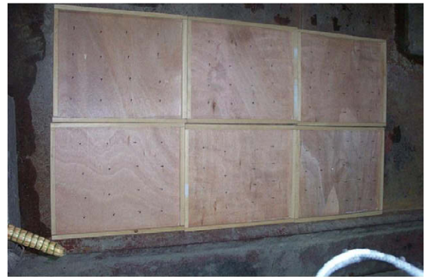
(b) specimen set with wooden formworks
